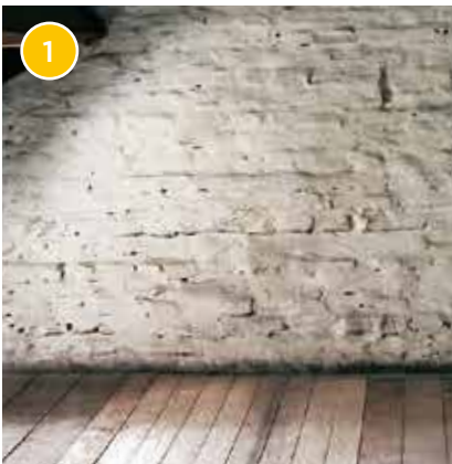
The substrate that you are covering with Rigidur flooring elements must not give or be elastic. And it must be dry and able to bear loads. First, prepare the substrate. In case of a wooden beam ceiling fasten loose boards, etc.
