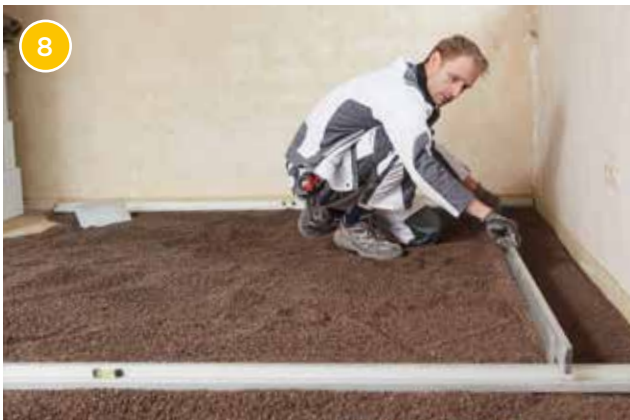
Smooth out and level the surface with a smoothing gauge over the levelling boards. Then remove the boards.
