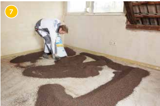
Raise two parallel banks at the desired levelling height, lay levelling boards on them and align the latter.
