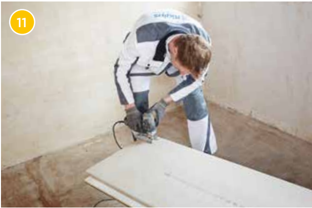
Cut the rebate edges off the first flooring element at the wall connections of the longitudinal and transverse side.
