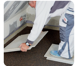
Laying the Flooring Elements on Rigidur levelling compound using "stepping stones"
