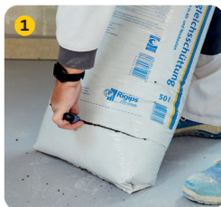
Cut the bag open at the bottom
