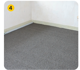
Flat surface of the bonded fill
