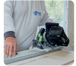
The rebate edge should be cut off where it abuts a wall
