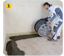
Spreading bulk material
