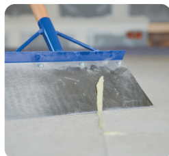
Knock off excess hardened adhesive
