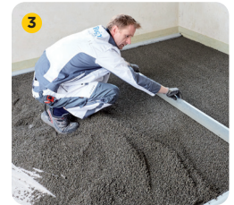
Smooth off using screed rails
